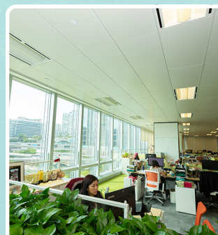
Sensor along with windows at head office and auto light off when exceeding 650 lux and during lunch hours
